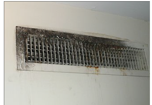
Finished attic air register
